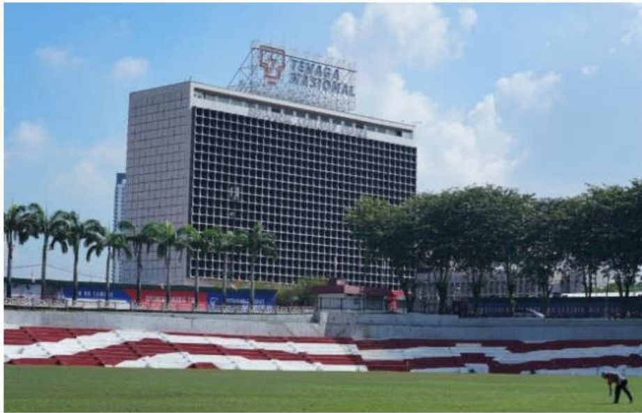
Sunway Construction Group Bhd's subsidiary has secured a RM781.30mil contract from Tenaga Nasional Bhd for the power giant's campus in Bangsar.
